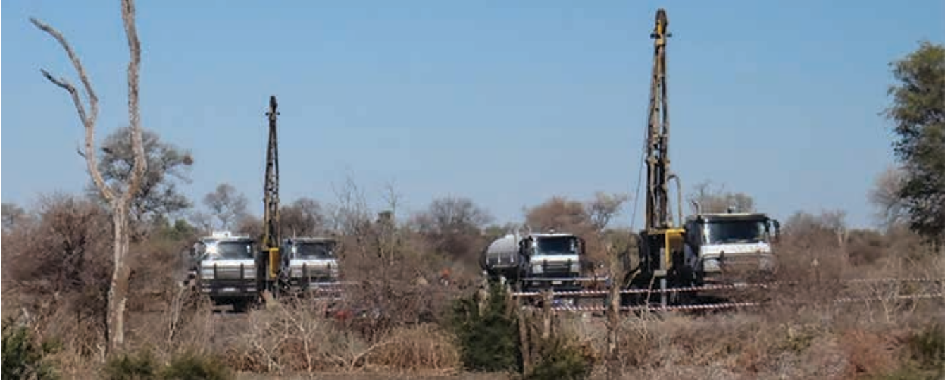
Drilling work at the XIF project.
